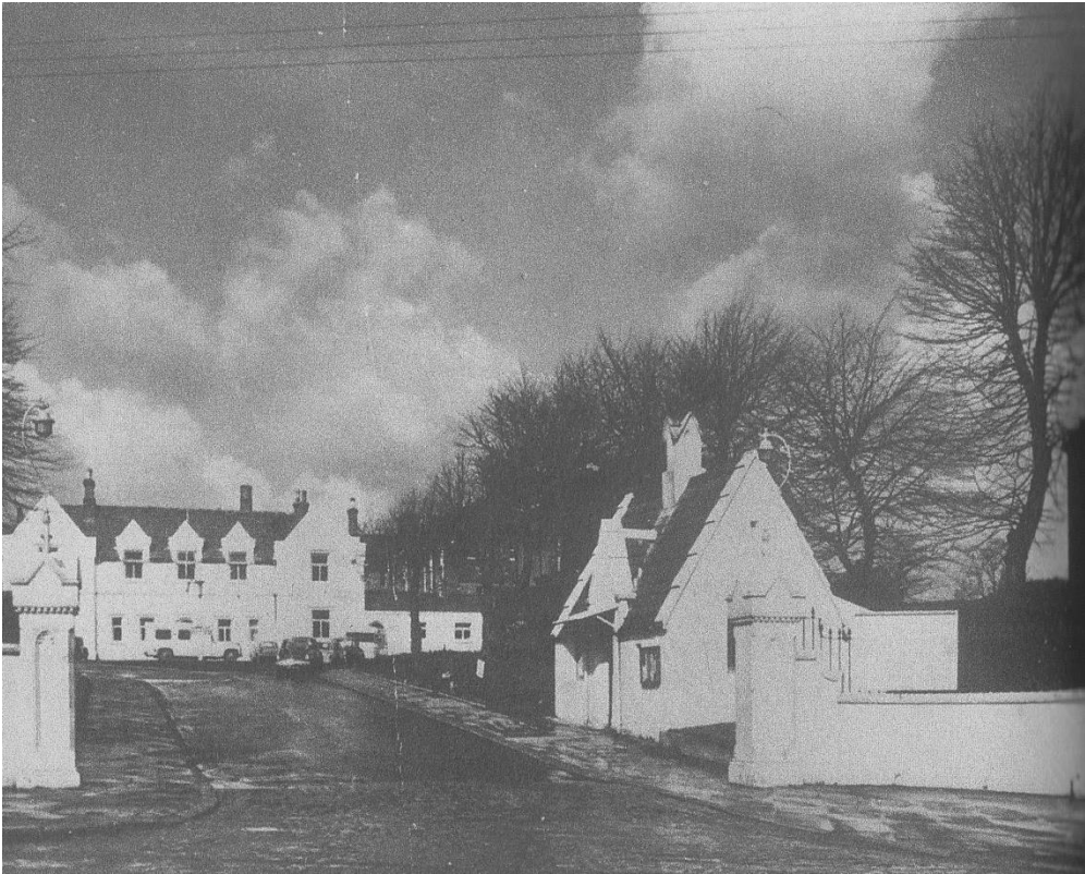
Original buildings of the work house
