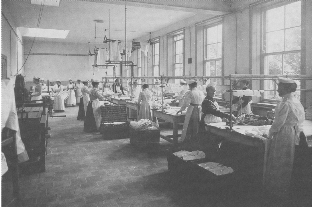
Laundry at Edgar House, Brunswick St, 1901
