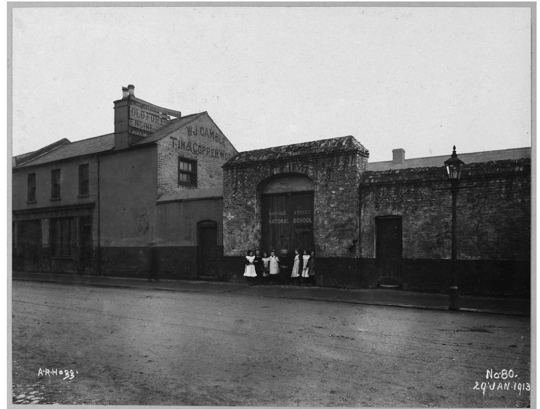
Barrack Street, National School, 1913
