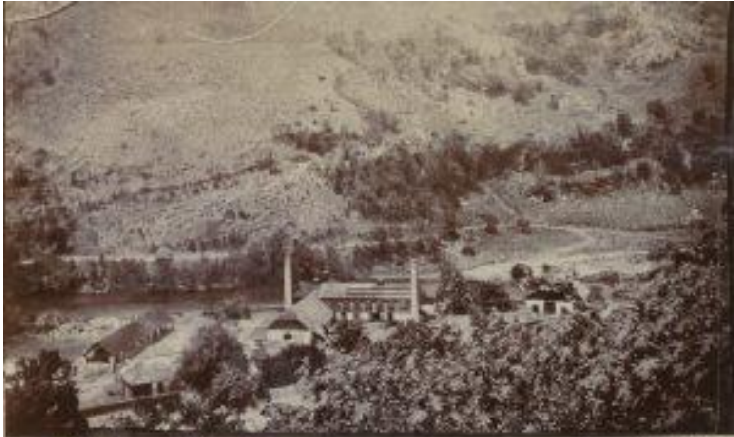
Hillsboro' Works May 1896 J. House
