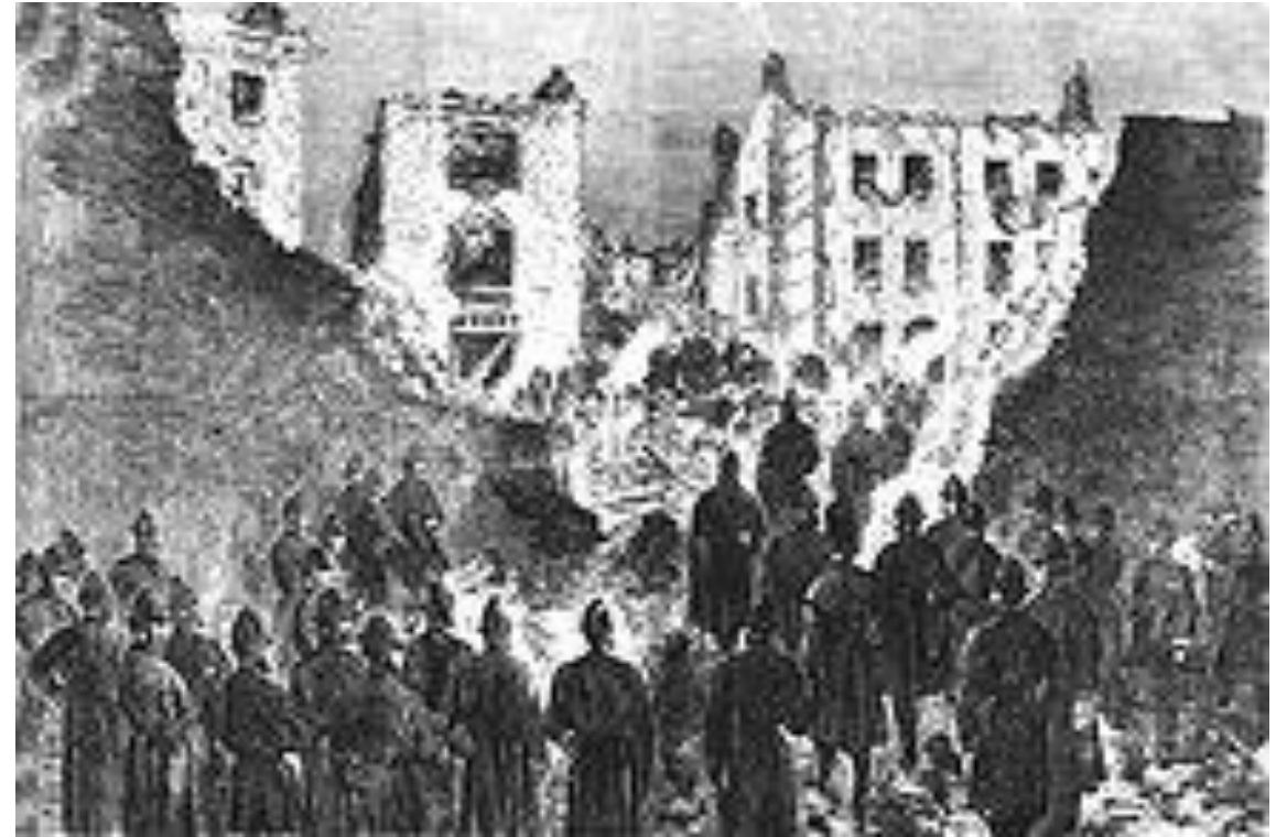
The House of Detention in Clerkenwell after the bombing; seen from within the prison yard
